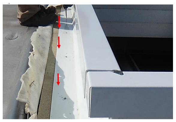
Fig. 30. Connecting the base to the roof with screws.
