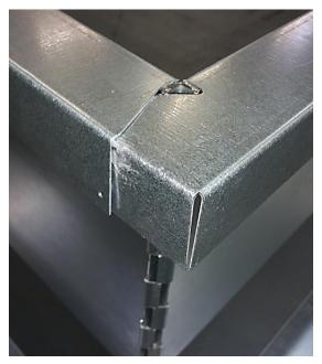
Fig. 25. Properly connected walls.
