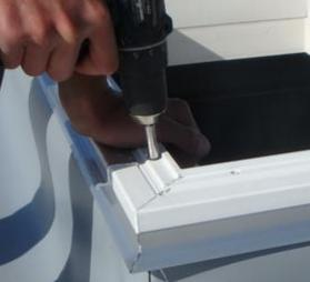
Fig. 35. Screwing the PVC top flange of base to the metal base.
