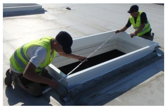
Fig. 29. Checking diagonals.
