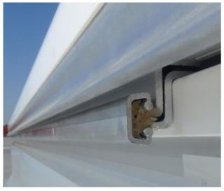
Fig. 43. Hinge connection mounted.
