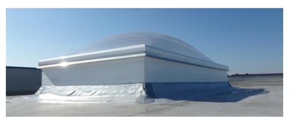
Fig. 19. Skylight / ventilation vent / roof hatch mcr ULTRA THERM after installation.
